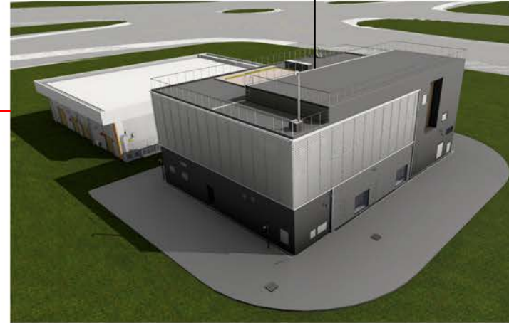
AFC Decontamination Facilities
