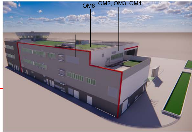
Airside Fire Station -Side view
